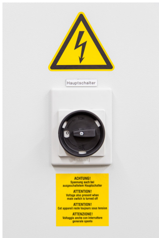
Figure 1: Main switch Control cabinet door
